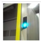
The traffic light system either has a sensor above the dock leveller that measures the presence of the vehicle or it is a wheel chock that detects the vehicle.
